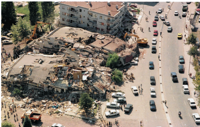
(a) Collapsed buildings in the aftermath of an earthquake.
